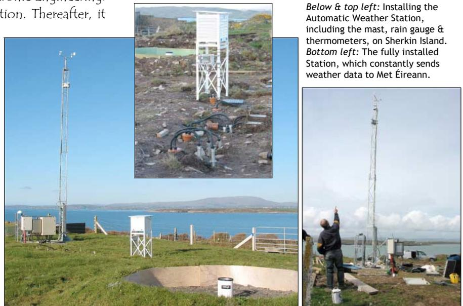
*Below & top left:* Installing the Automatic Weather Station, including the mast, rain gauge & thermometers, on Sherkin Island. *Bottom left:* The fully installed Station, which constantly sends weather data to Met Éireann.
