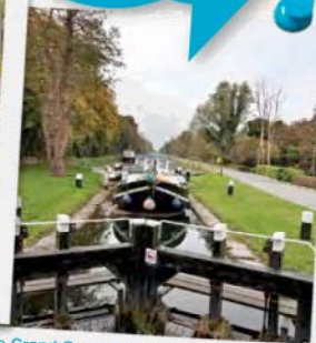
The Grand Canal 30th Lock Located on the Grand Canal the 30th Lock is operated manually through the use of a lock key
